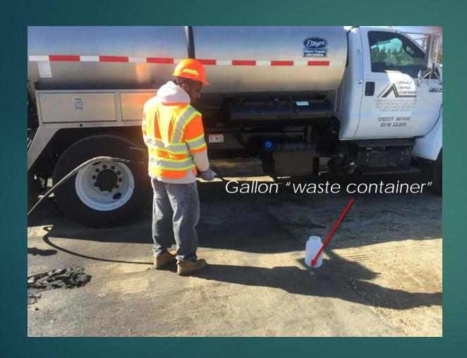
Allow minimum one gallon to flow into "waste container" and discard.
