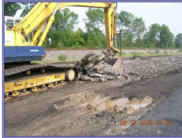
Asphalt Pavement Removal
