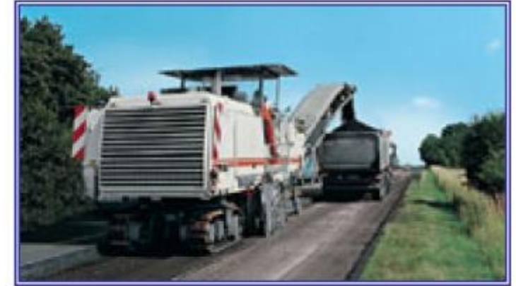
Pavement Milling
