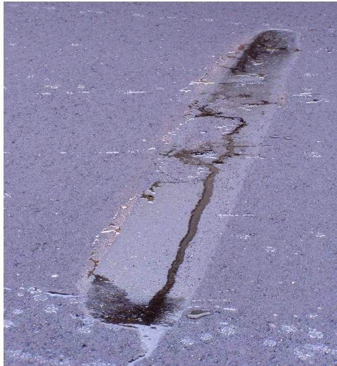
“Birdbath” from roller stopping on hot mat
