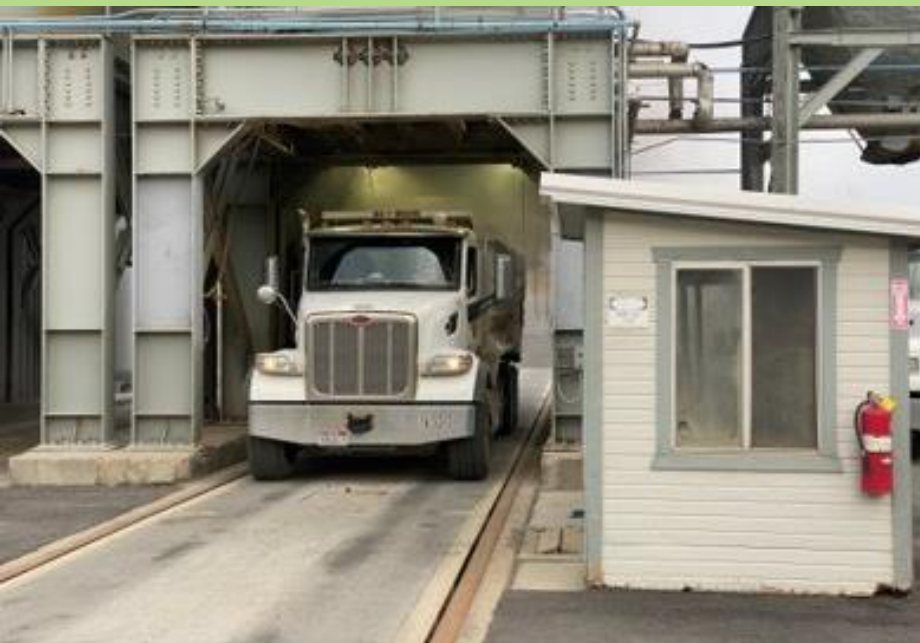
Smoke – Standard Hot Mix Asphalt at 315F
